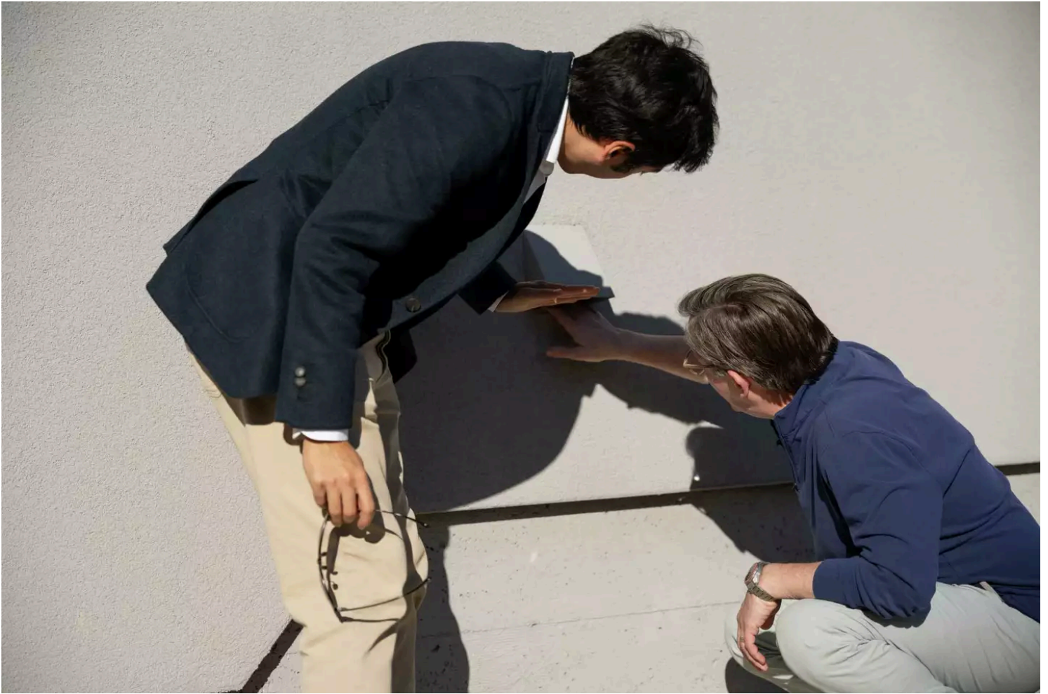
Mercury Insurance President Victor Joseph, left, and Roy Wright, CEO of the Insurance Institute for Business and Home Safety, inspect a newly constructed home in Paradise in Butte County during a tour of the town's rebuilding efforts. Florence Middleton/Special to the Chronicle
