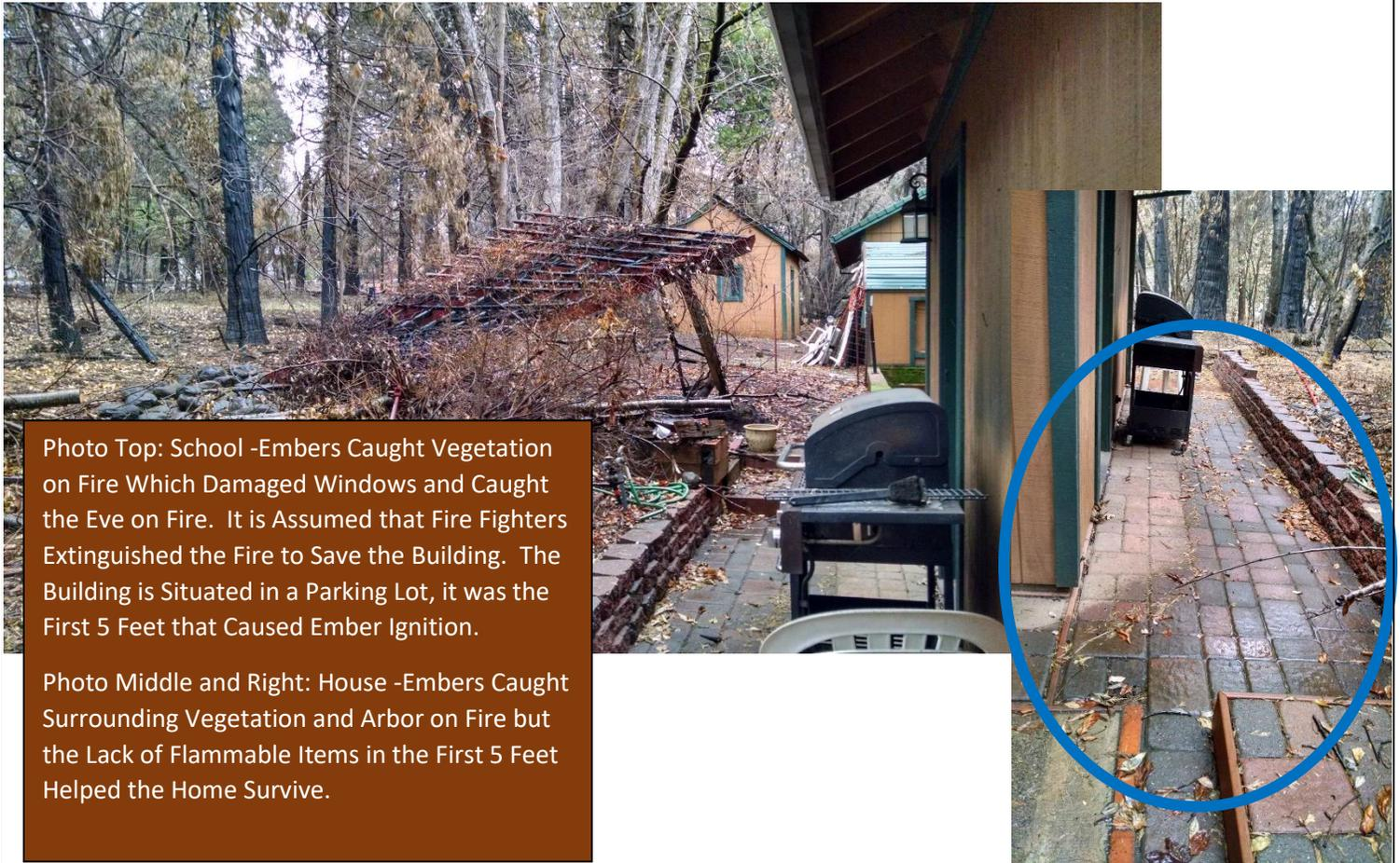
Photo Top: School -Embers Caught Vegetation on Fire Which Damaged Windows and Caught the Eve on Fire. It is Assumed that Fire Fighters Extinguished the Fire to Save the Building. The Building is Situated in a Parking Lot, it was the First 5 Feet that Caused Ember Ignition.
